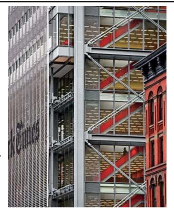
The square cross floor plan design is to expose the interior to as much daylight as possible. Although the building is fully glazed allowing direct sunlight to enter, which causes problems for most buildings, the second skin consist of a sunscreen of white ceramic rods to minimize these problems. It reduces heat gain and too much light, while also forming a connection between the building and the city.
